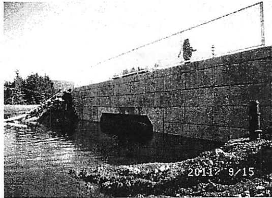
Klawock lagoon causeway before and after the breach restored tidal flushing and fish access; Photos by TNC
