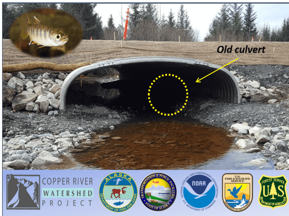
Figure 3. Fish passage culvert replacement in the Copper River Basin depicting the location of the old culvert (yellow dotted circle) with the new culvert. Photo credit: CRWP.
