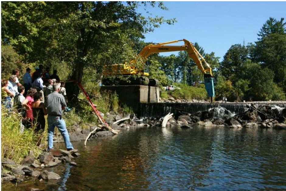
Brownsville Dam Removal, Oregon. Photo credit: NOAA
