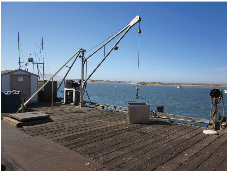
Photo: 2,000 pound stainless steel offloading hoist at the 1099 Embarcadero facility.
