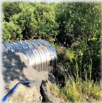
Fish passage restoration on the Buskin River in Kodiak, AK.
